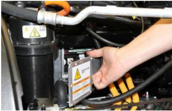
Removing the lid for high voltage connections
